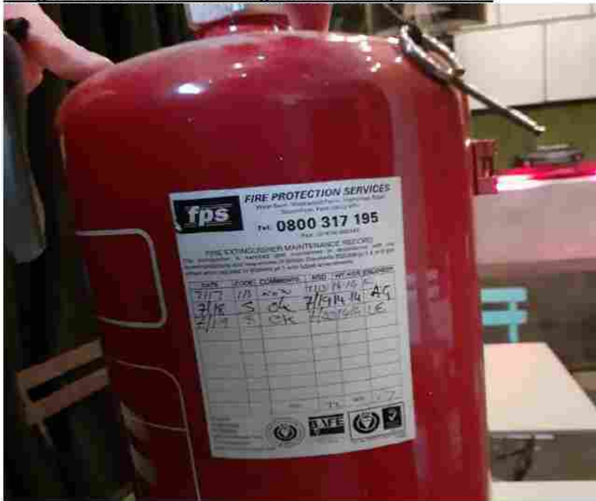
Image 2 -Out of date fire extinguishers last inspected 2019
