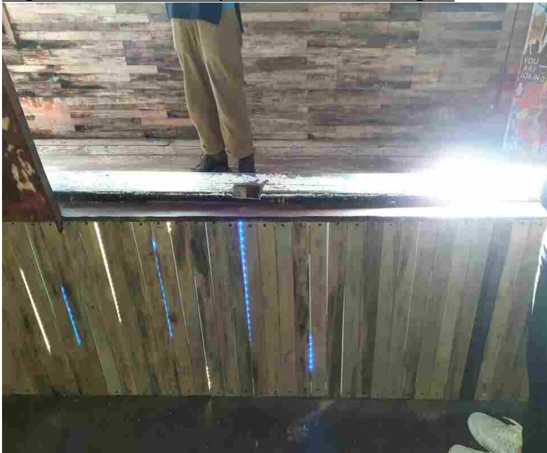
Image 6 – Low wall not secured to prevent customers from climbing over
